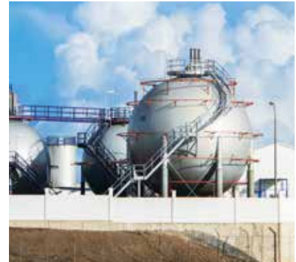
Part of a desalination plant
